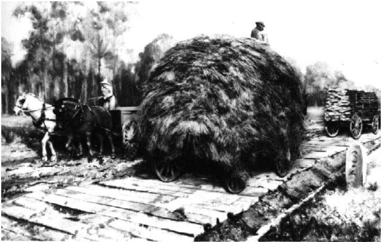
Taking goods to market on a plank road, in this case the Leesburg Pike, a toll road.
